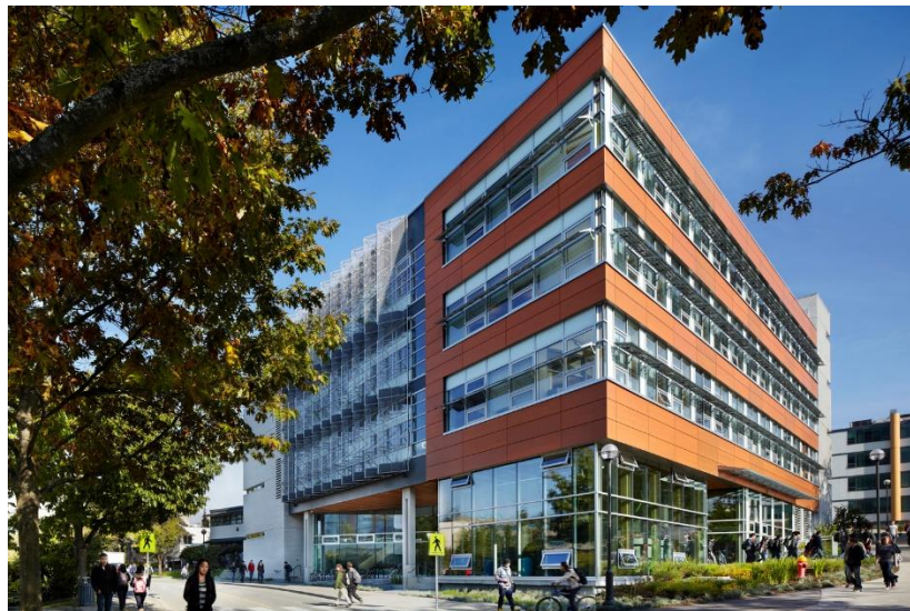
Figure 2.3: Image showing the Facade of the CIRs (Source:
