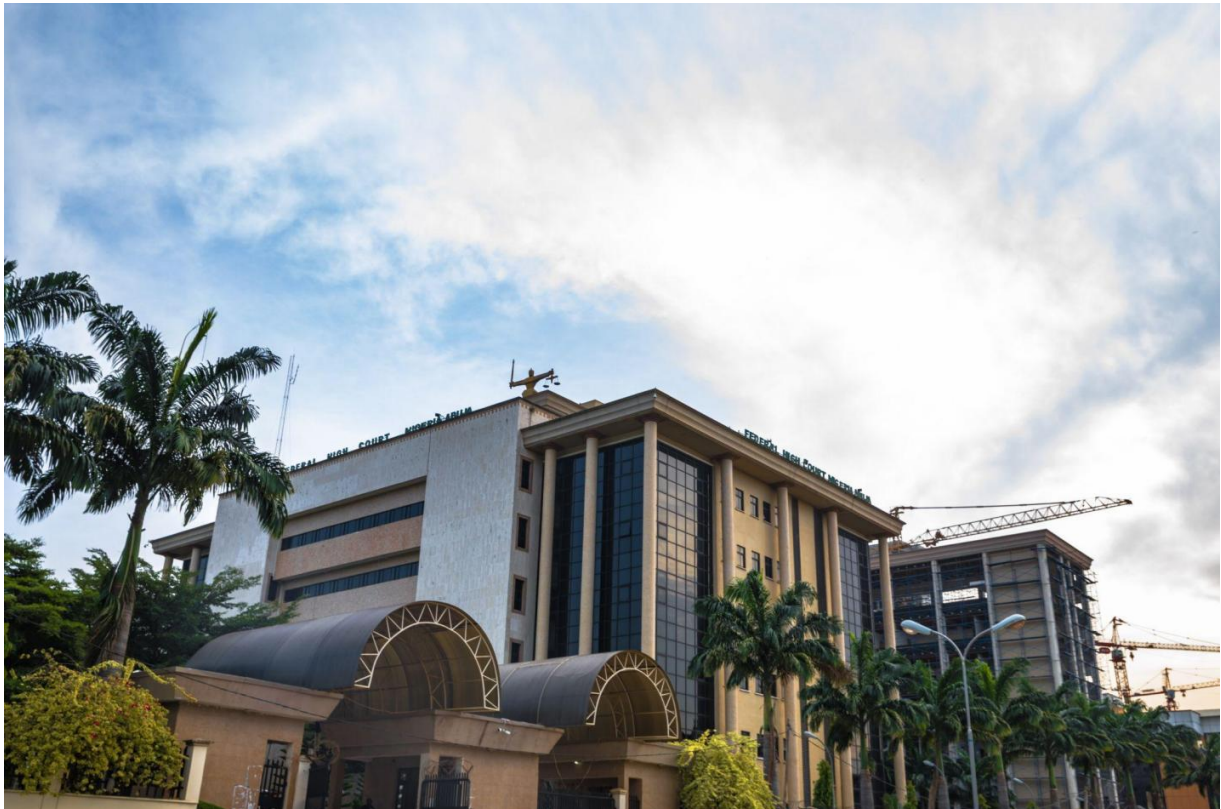
Plate 2.1: Image showing the Facade of the Federal High Court Complex, Abuja (Source: Wikipedia, 2026)
