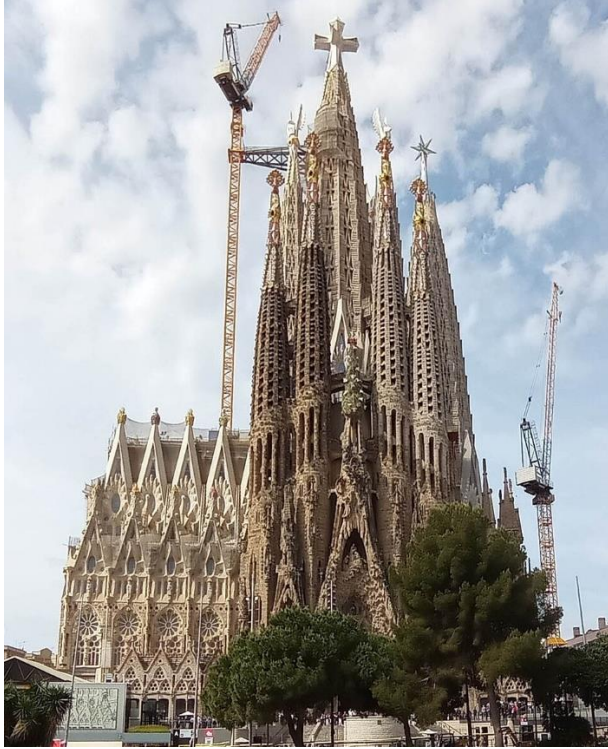
Plate 2.11: Ventilated view of the outside of Sagrada Família, Barcelona, Spain.
