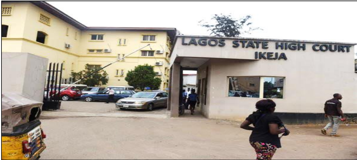
Plate 2.3.3: Lagos State High Court, Ikeja (detailed view of the entrance of the court)(Source: Wikipedia commons, 2026)
