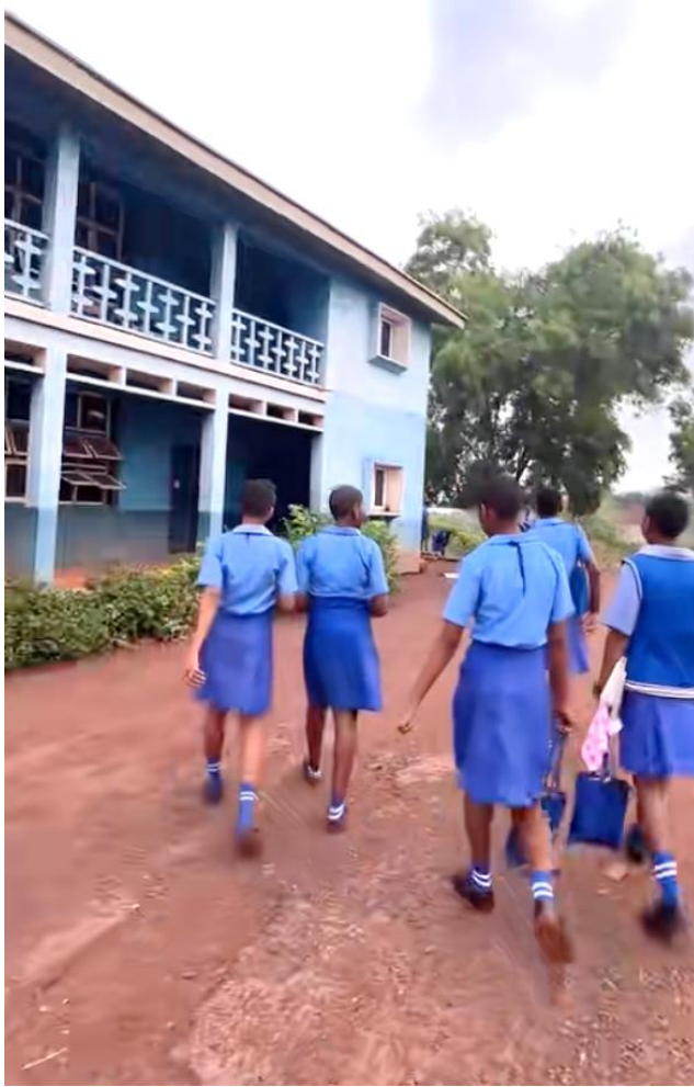
Figure 2.8 Showing the school building ( sources: field work)
