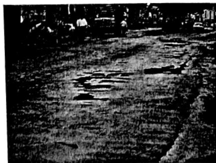
Plate 2. Irregular Cross and longitudinal slopes resulting in ponding.
