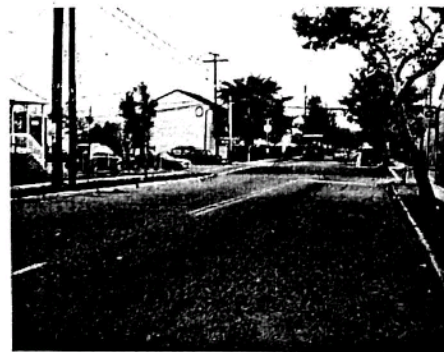
Plate1. Street with convex crown and slope.
