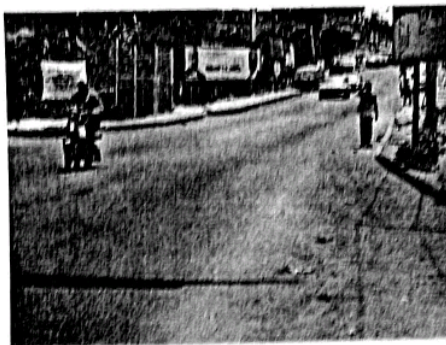
Plate 6. University Road – siltation and non-evacuation of silt from edges.
