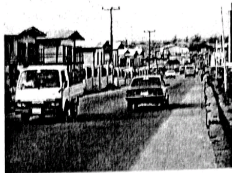
Plate 5. Aswani Road exhibiting fair longitudinal slope with siltation along the edges.
