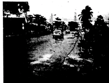
Plate 3. Ponding resulting from roller-coaster slopes.
