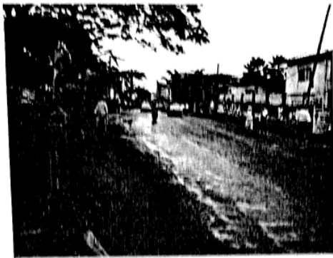
Plate 4. Street edges at higher levels than the center of street.
