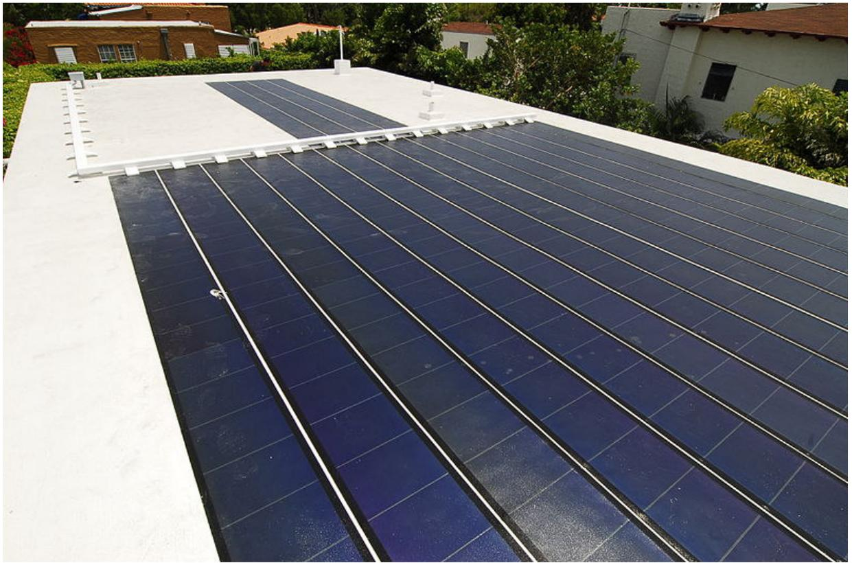
**Figure 7b:** This thin-film laminates on rooftops
