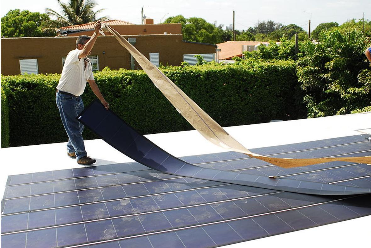
**Figure 7a:** This is a thin-film silicon laminates being installed onto a roof.
