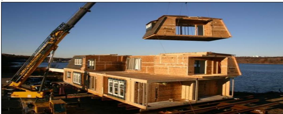
**Figure 3: Example of Modular Construction**
