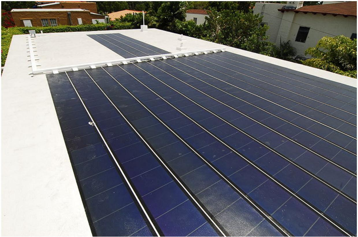
**Figure 7b:** This thin-film laminates on rooftops
