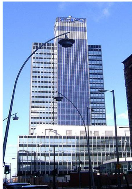
**Figure 7c:** This is the CIS Tower in Manchester, England was clad in PV panels at a cost of £5.5 million. It started feeding electricity to the National Grid in November 2005.
