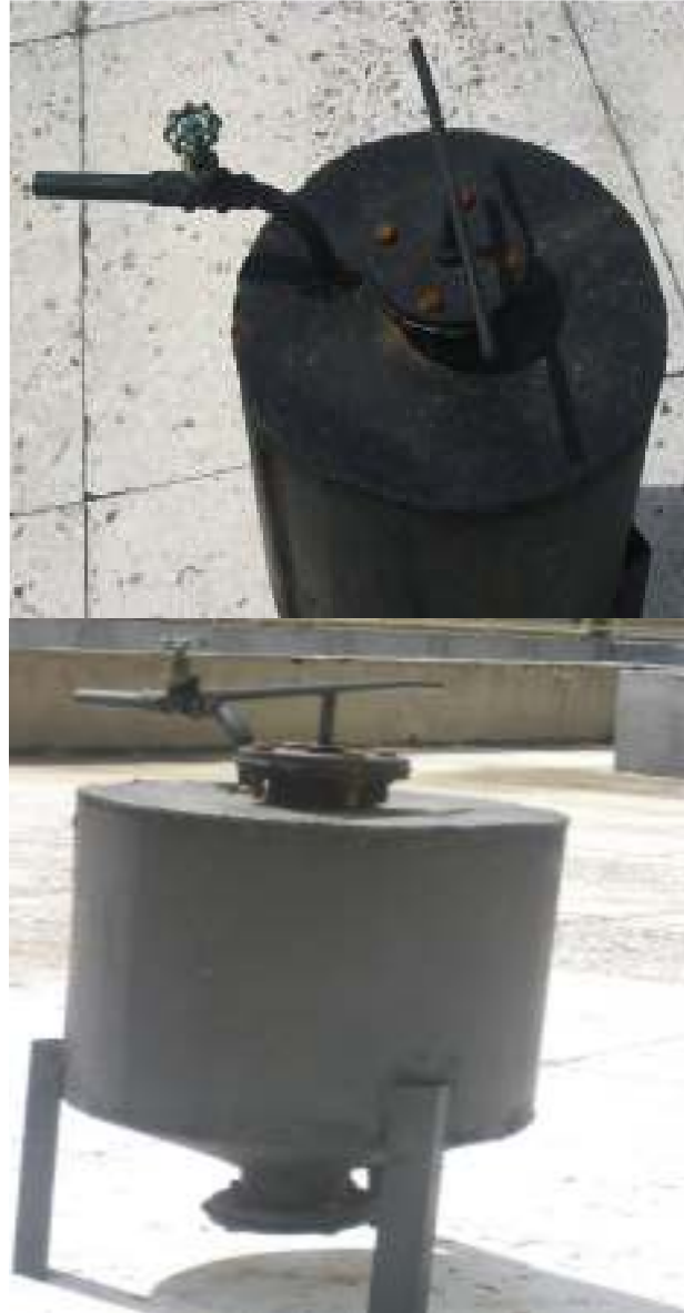
Fig. 1: Picture of constructed biogas digester.
